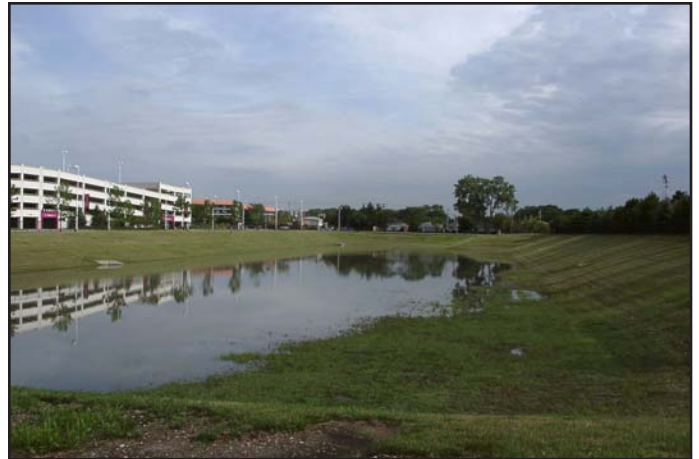
Dry detention pond - Picture courtesy of Aaron Volkening, P.E.
