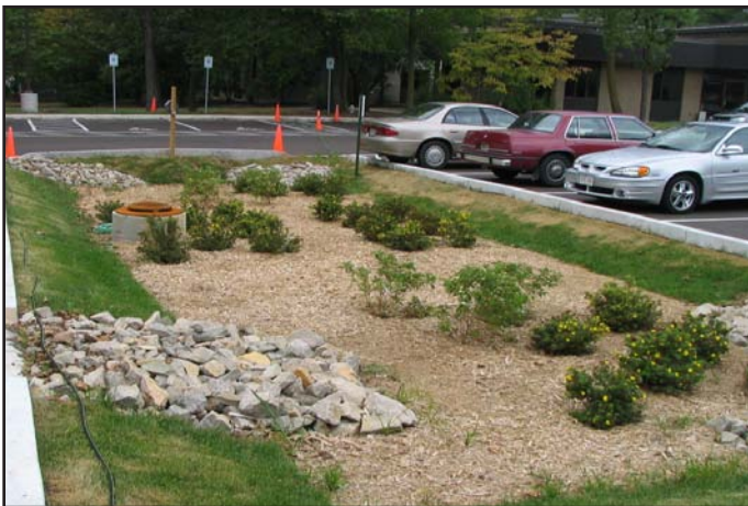
Bioretention area/rain garden - Picture courtesy of Aaron Volkening, P.E.
