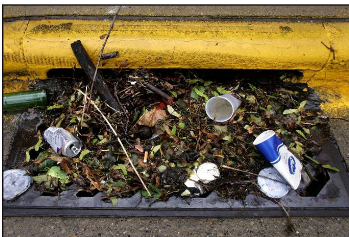
Grates can filter trash and debris from stormwater - Picture courtesy of Aaron Volkening, P.E.
