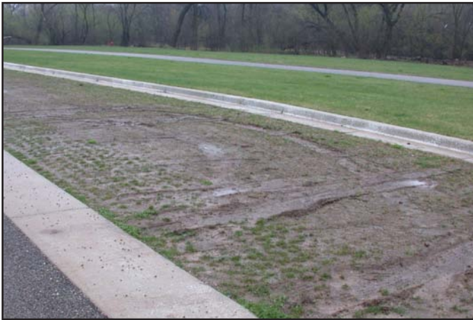
Porous pavement - Picture courtesy of Aaron Volkening, P.E.
