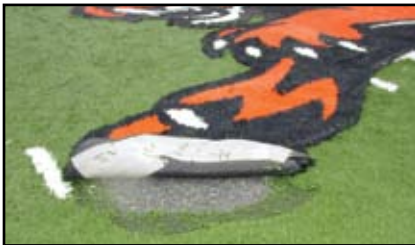
Installation of a special logo on a synthetic field. Photo: Darian Daily
