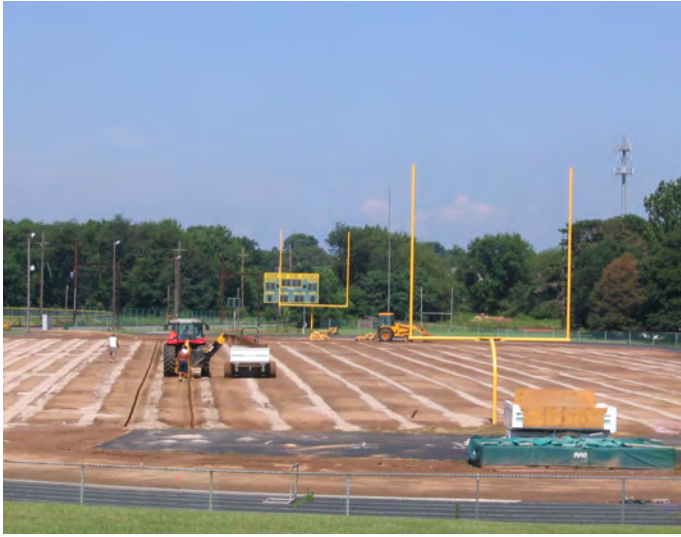
Installation of drainage pipe system - Photo courtesy of Doug Linde, Ph.D.
